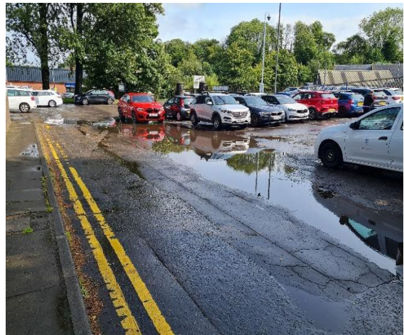
Photo 22: Tarmacadam surfaces to car park/road in poor condition.
