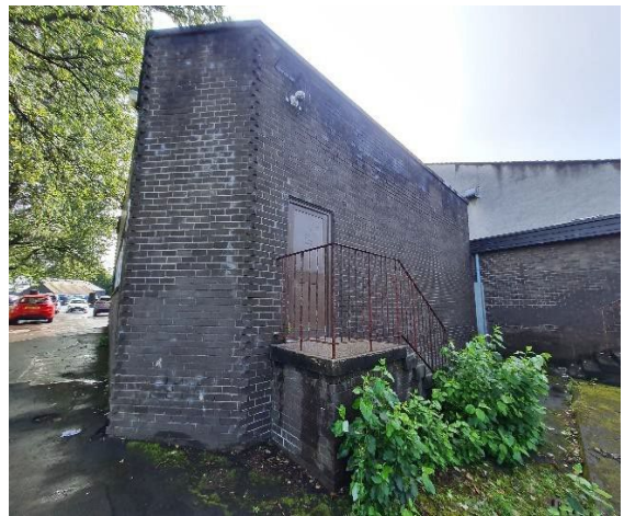
Photo 24: External surfacing suffering from breakages and excessive vegetation.
