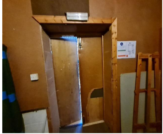
Photo 20: Internal doors typically poor condition.
