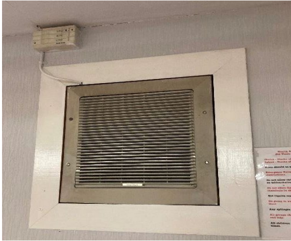
Photo 25: Wall-mounted axial extract fan in Hall.
