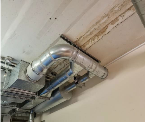
Photo 19: Cracks and water ingress evident to ceiling.
