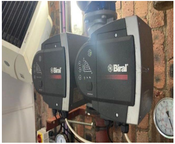
Photo 41: Twin Head Pump Set
