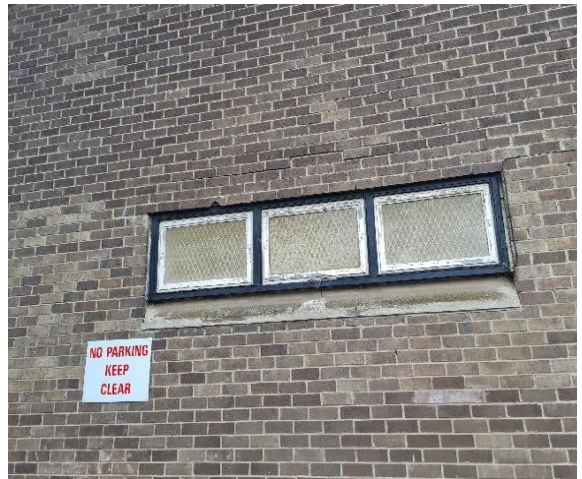
Photo 10: Original timber windows, stepped cracking above around lintel position.
