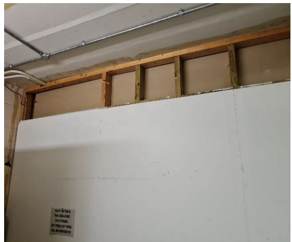
Photo 18: Recent partitions erected without correct compartmentation detailing.
