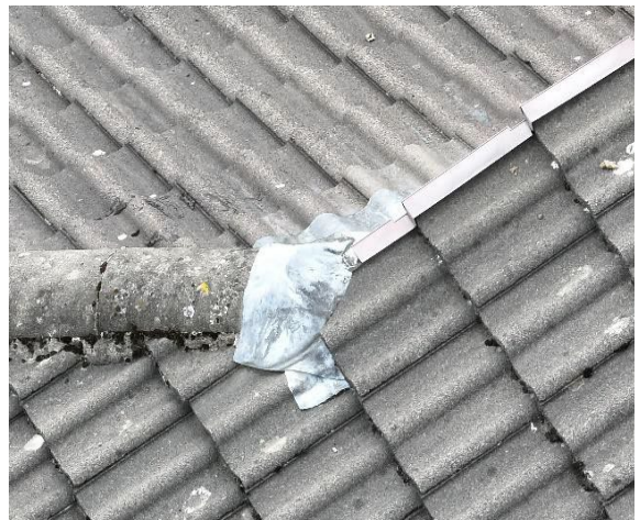
Photo 6: Poor detailing at roof junctions.
