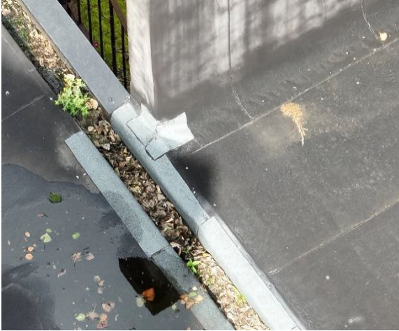
Photo 7: Felt covering to flat roofs with some patch repairs evident.
