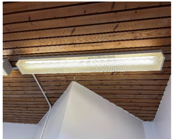
Photo 34: Example of a surface mounted linear fluorescent luminaire.
