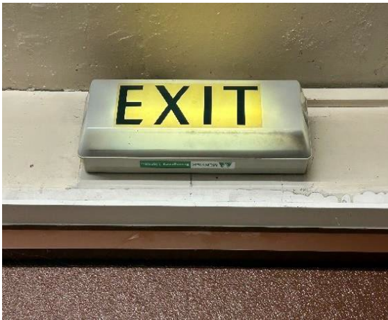
Photo 31: Example of fluorescent emergency lighting bulkhead.
