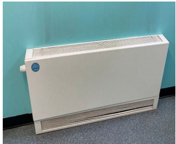
Photo 43: Stelrad LST Radiator in Male Toilet
