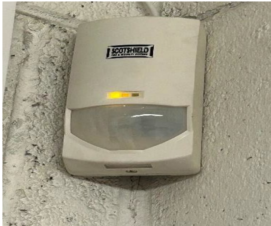
Photo 27: Typical PIR sensor found building wide.
