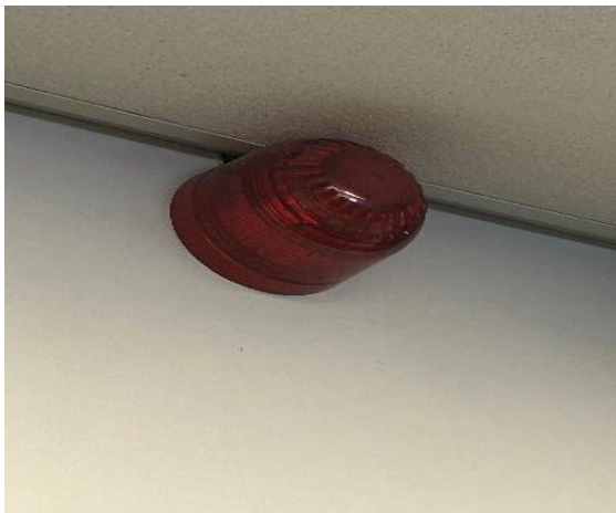
Photo 29: Typical example of sounder found building wide.
