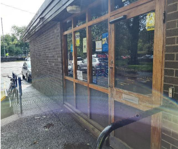
Photo 13: Front entrance, external doors in poor condition.
