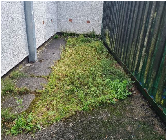
Photo 23: External surfacing suffering from breakages and excessive vegetation.
