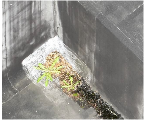
Photo 4: Flat roof outlet blocked.
