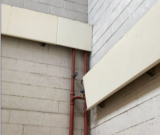
Photo 44: Wall Mounted Radiant Panels in Main Hall.
