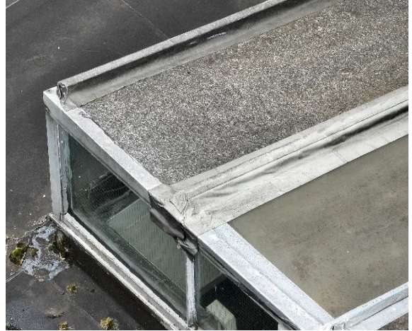
Photo 8: Rooflight in poor condition with possible wood wool slab/panel infill.
