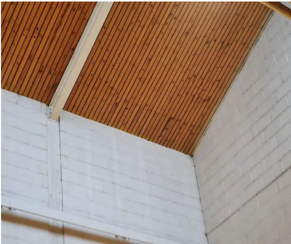
Photo 15: Isolated areas of timber panelling loose at high level
