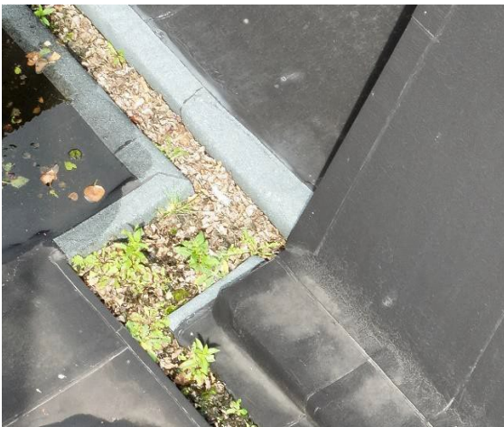
Photo 5: Flat roof with gutters choked.
