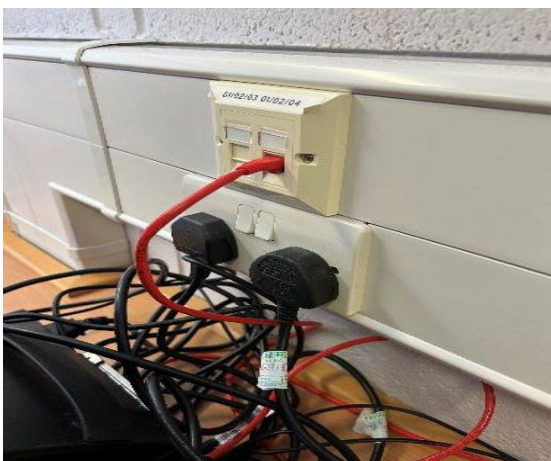
Photo 35: Example of typical dado trunking, located in IT Suite (033).
