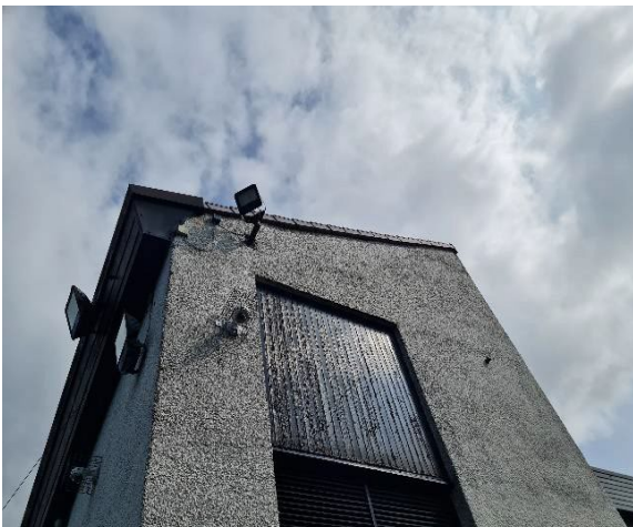
Photo 11: Large areas of render have been replaced, some areas older style.
