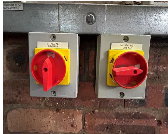
Photo 26: Typical example of isolators found building wide.
