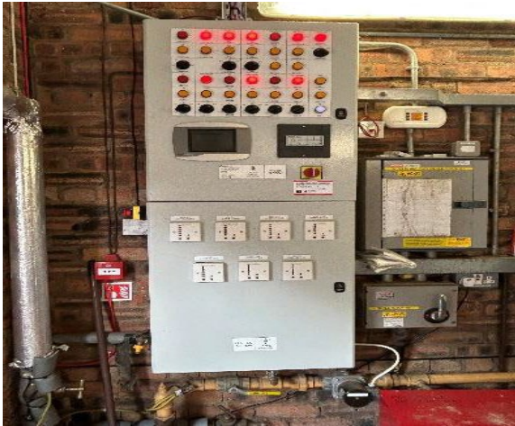
Photo 25: Building management system located in the Boiler Room (048).
