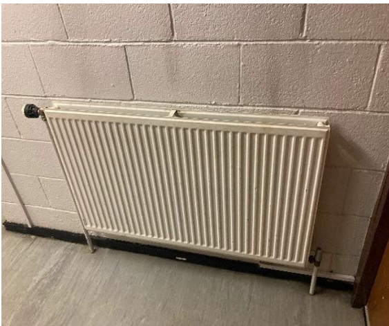
Photo 42: Steel Panel Radiator with TRV
