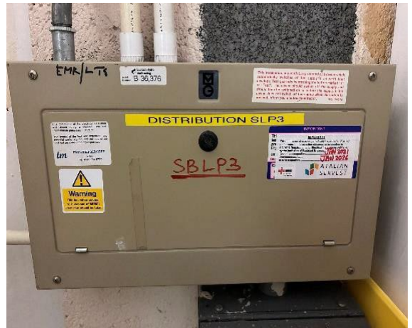
Photo 28: Example of distribution board out with its lifespan located in Store (010).
