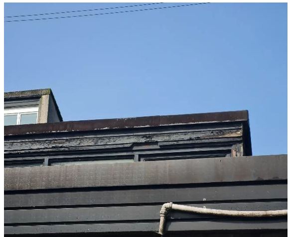
Photo 12: Defective facias and overflow pipe from gutter installed.
