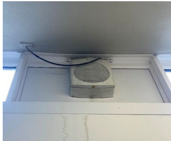
Photo 24: Wall-mounted extract fan in Male Toilet.
