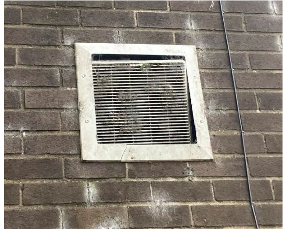
Photo 26: Exterior of axial extract fan in Hall.
